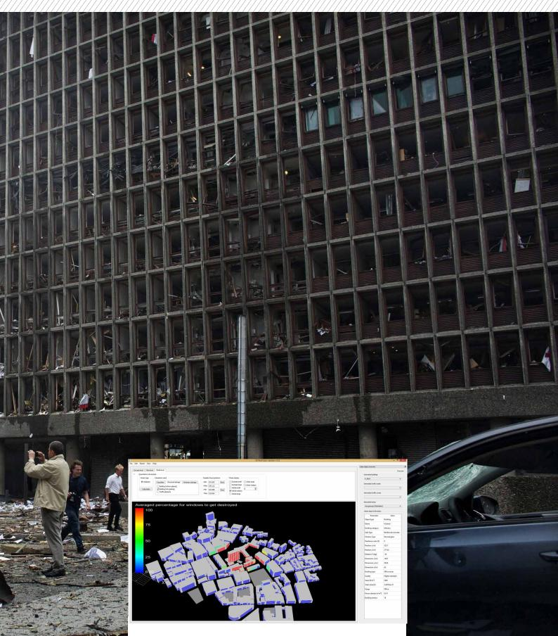
The picture shows a screenshot of the VITRUV software tool which was used to analyze the most probable locations for an attack in the government quarter of Oslo comparable to the one that really happened as well as its damaging effects on the surrounding buildings.
